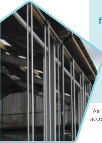
Air inlets can be controllable according to weather conditions
